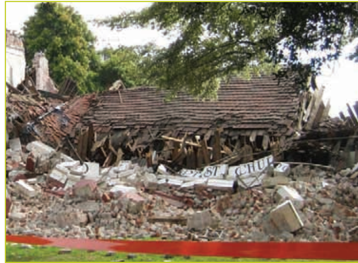
Unreinforced masonry building after the 22 February Christchurch earthquake
